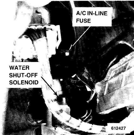
Figure 2 - LH Side of Evaporator Housing
