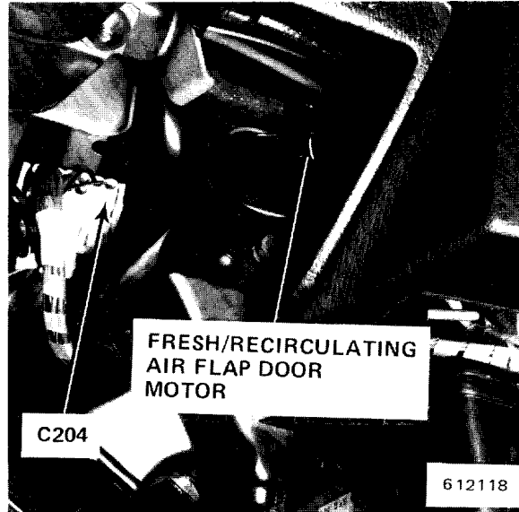
Figure 4 - LH Side of Evaporator Housing
