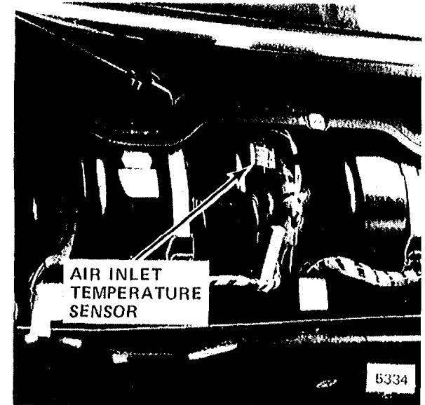
Figure 5 - Under Center of Fresh Air Intake Cowl
