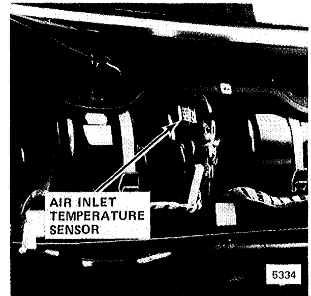
Figure 5 - Under Center Of Fresh Air Intake Cowl
