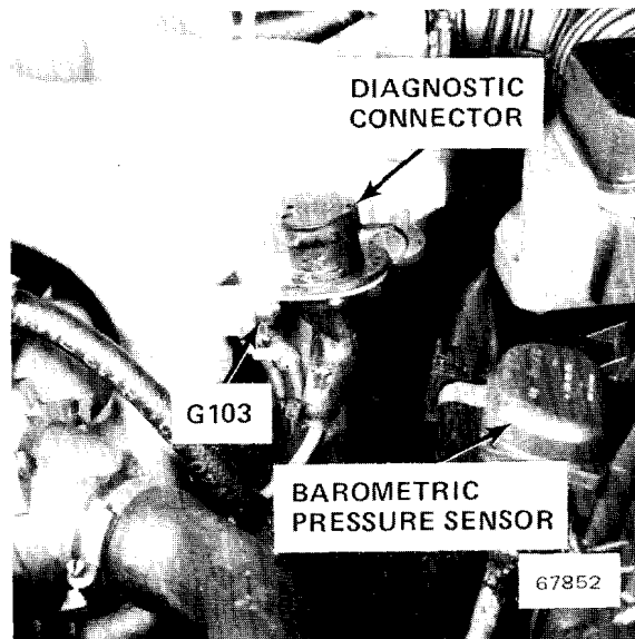
Figure 4 - LH Front of 528e Engine Compartment
